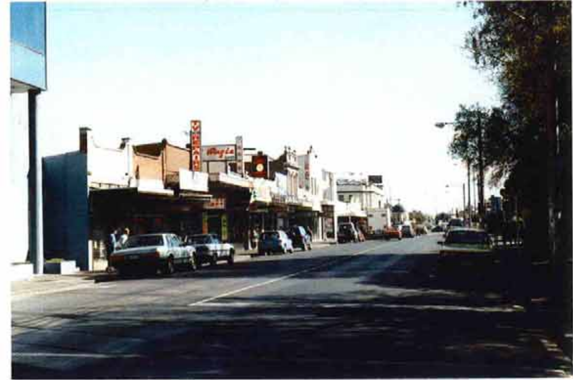
BARKLY STREET WITH BUNDLED POWER AND CONSOLIDATED POLES
