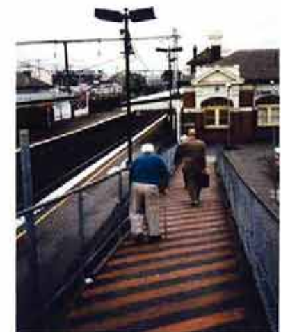
Pedestrian ramp Footscray Railway Station
