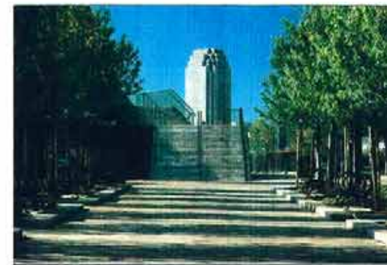
Pedestrian steps & ramps linking station platforms to be integrated into the square design
