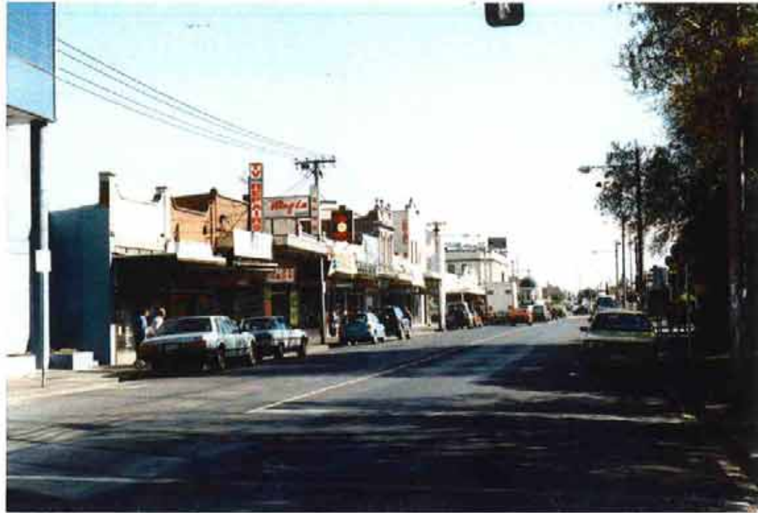
BARKLY STREET - EXISTING CONDITIONS
