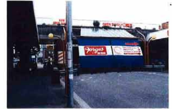
Existing bridge & road closure obstructs views
