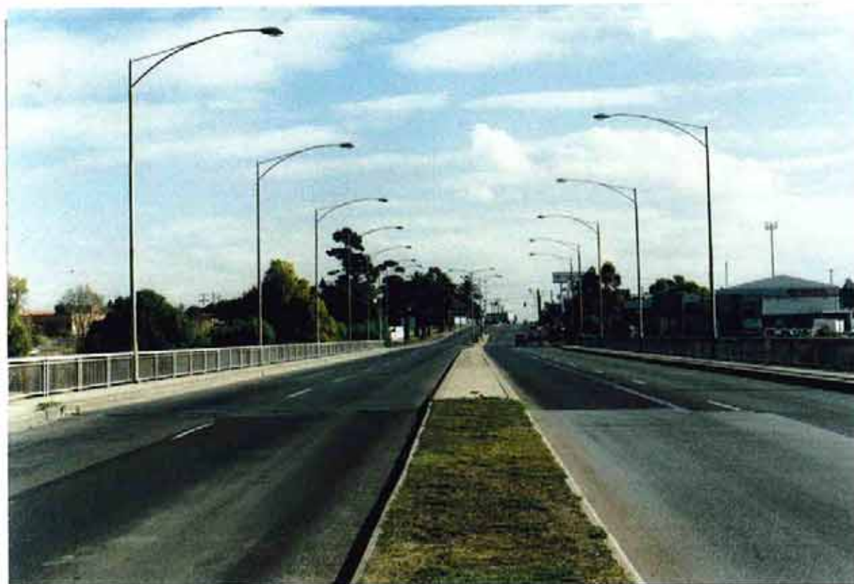
DYNON ROAD LOOKING WEST TO FOOTSCRAY - EXISTING CONDITIONS
