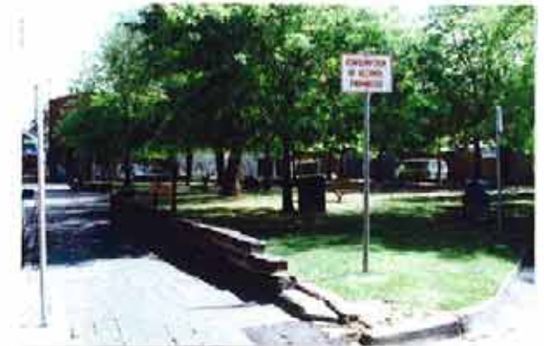
Existing low wall in poor condition & prevents easy pedestrian access into the square
