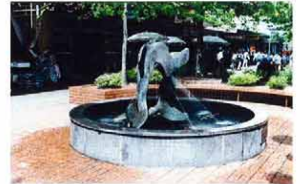
Existing fountain - oversplash problems
